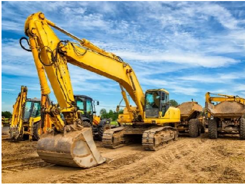
Figure 2 Machines on construction sites use plenty of simple machines to operate
