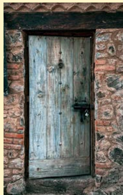
Lintel above door © moran
