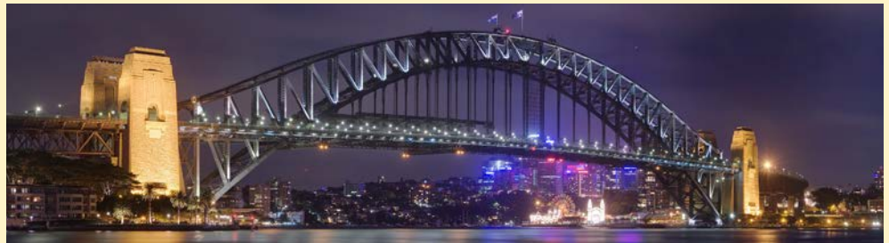
Sydney Harbour Bridge © Roantrum
