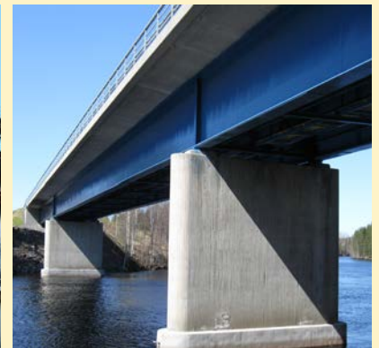
Steel beams supporting a bridge ©Ahmaskoski
